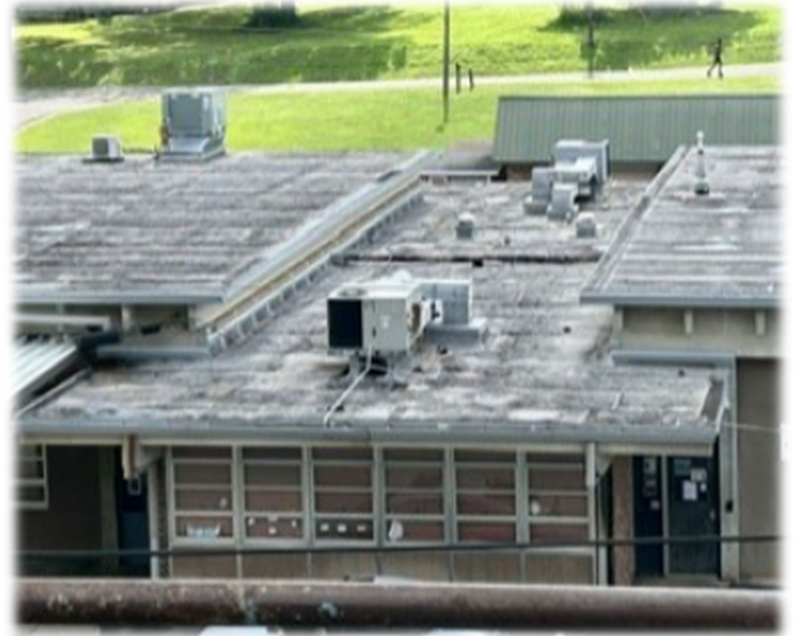
Gadsden State Roof and Gutter Replacement Project
