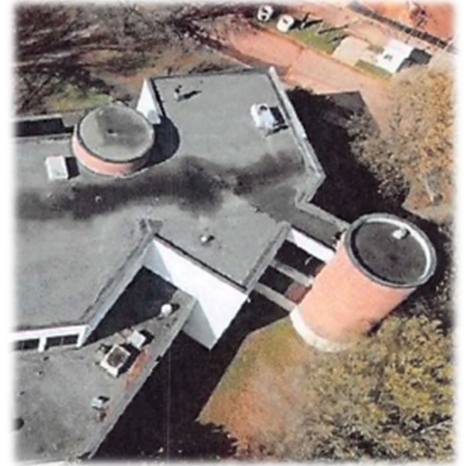
Lawson State Roof Replacement Project
